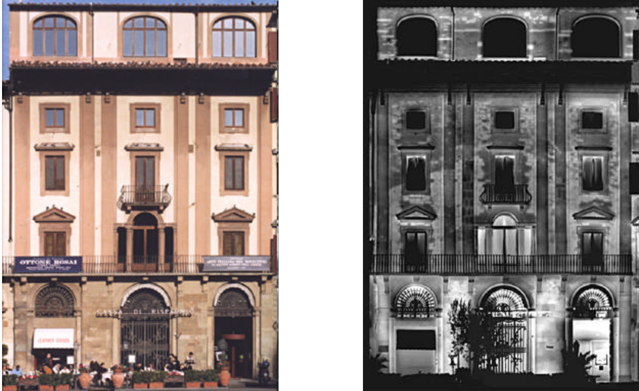
Figure 3: Thermographic inspection of a building.
